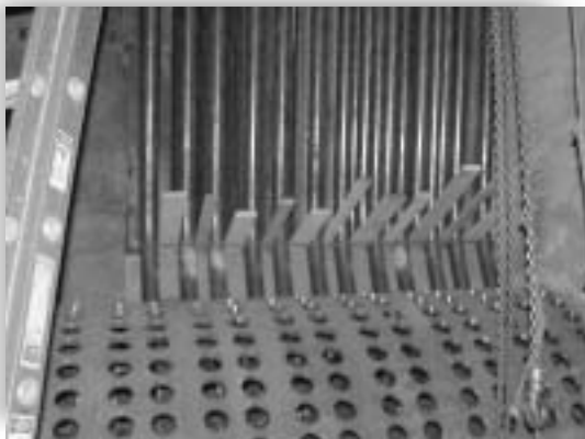
New tubes are inserted in a steam drum.
