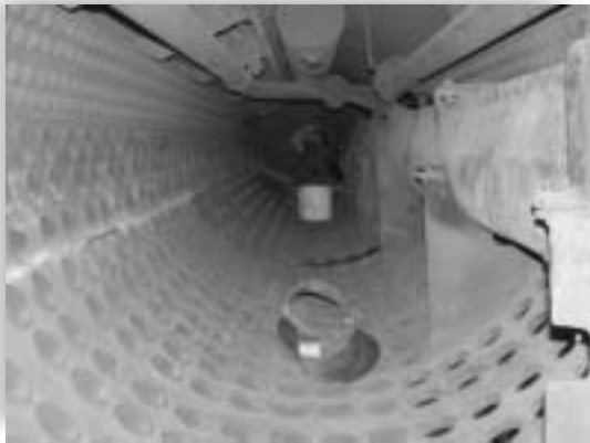
The inside of a steam drum is refurbished.
